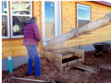
Steps poured, front, back & garage
