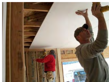
Interior of Garage is sheetrocked
