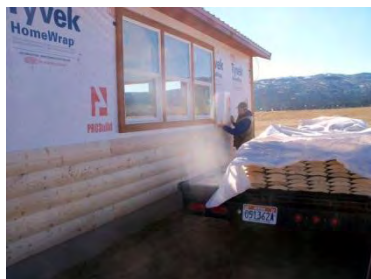
Siding on Garage
