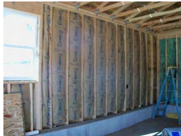
Interior of Garage Insulated
