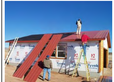
Metal Roof onto Garage
