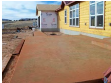
Front Porch & Sidewalk
