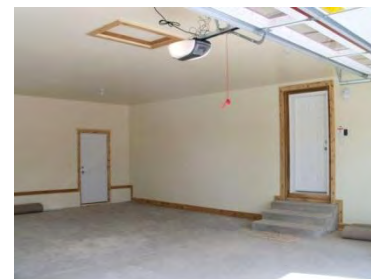
Interior Garage trimmed and Caulked
