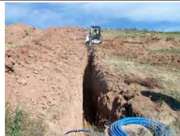
Trenching for the water line
