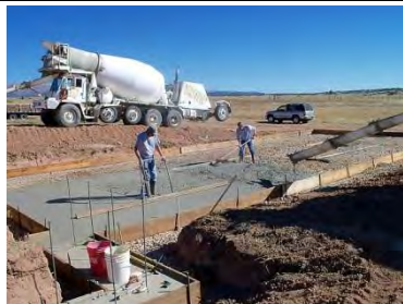
Footers and Foundation
