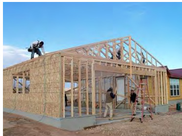
Framing for the Garage
