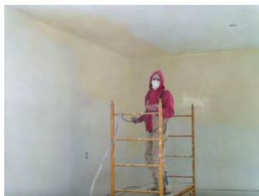
Garage Interior Painted
